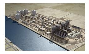
sulfur coal that is less desirable is deliberately burned in this plant because the sulfur is used to manufacture sulfuric acid.
